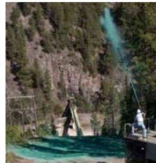
Figure 8: Hydroseed solution applied in Kirk Gulch. A pipeline on the bridge was installed in Fall 2010 to transport water from Grizzly Gulch tailings dam to the wastewater treatment plant.
