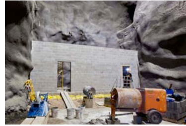
Figure 6: Infrastructure Tech Mike Oates standing in the doorway (right) of one partially constructed "counting room," where radioactivity of experiment components will be tested
