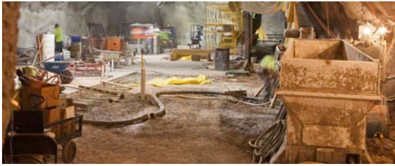
Figure 8: Work progresses at Transition Cavern
