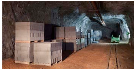
Figure 4: Concrete blocks stored in the chiller cutout awaiting use in construction of the Davis Campus
