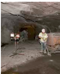
Figure 2: C-TEC and Sanford Lab personnel apply shotcrete on 4850 Level
