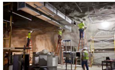
Figure 8: Tessier's Inc. crew hangs ducts in the Transition Cavern
